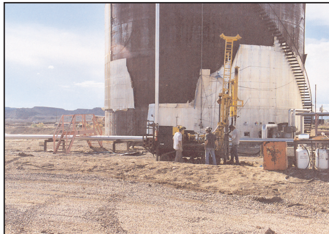
Installation of monitoring wells at site in Fruita, CO.
