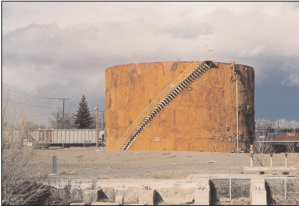
Aboveground storage tank at Alamosa Power Plant site.
