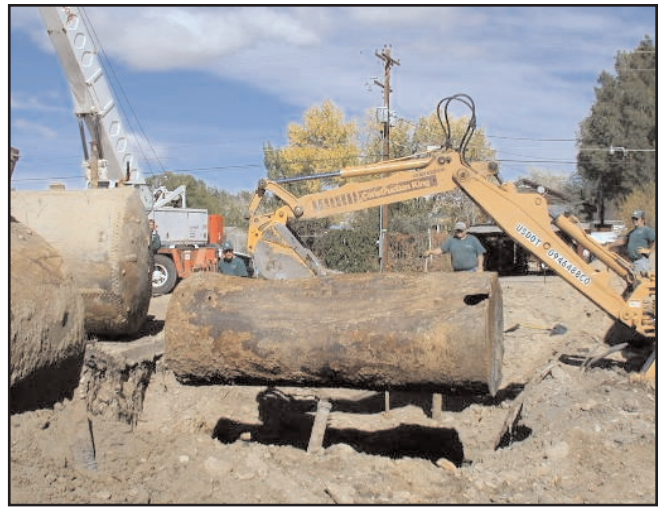
Underground tank removal at Galaxy site.
